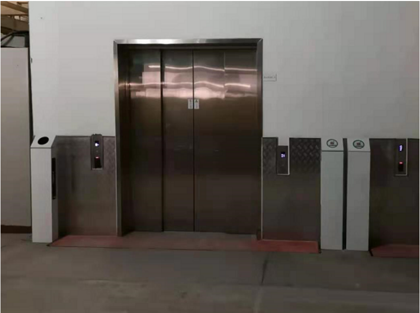
Erecting Identification Device
